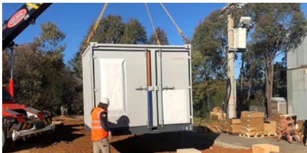
The Yackandandah battery is craned into position. Image: TRY
